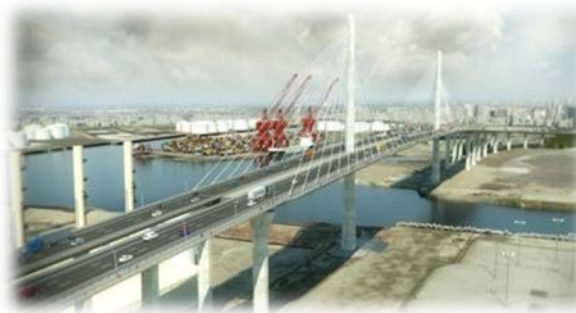
Gerald Desmond bridge in Los Angeles (USA)
