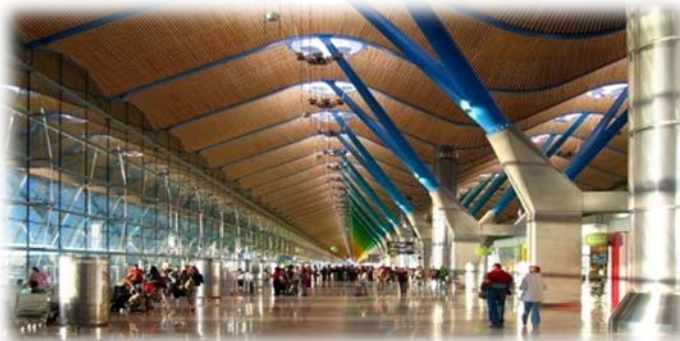
Madrid Barajas Airport Terminal 4, the largest civil engineering project in Europe, which received the International RIBA European Award 2006
