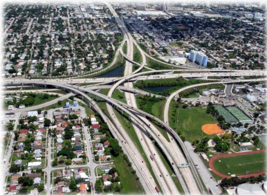
I-95 Miami Express in Florida (US), won the Best in Construction 2010 award and America's Transportation Award 2009
