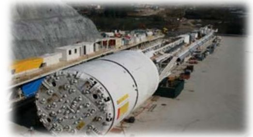
Southern ring road in Prague (Czech Republic)
